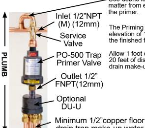
Use debris loop to ensure foreign matter from entering directly into the primer.
